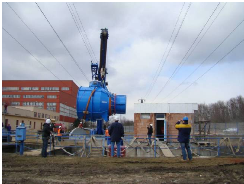
Kaplan turbine installation
